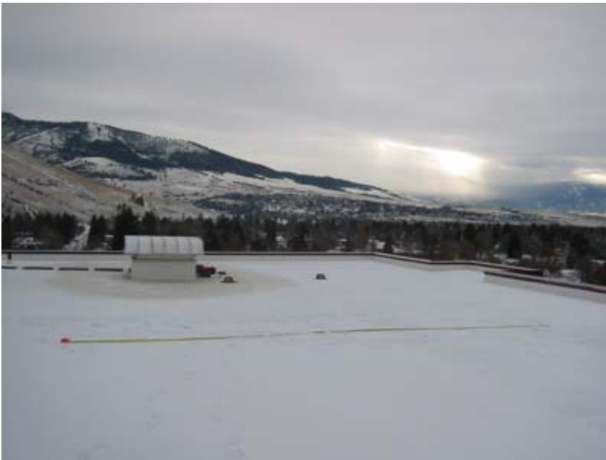
Photo #4: Skaggs rooftop with 20' on the tape.
